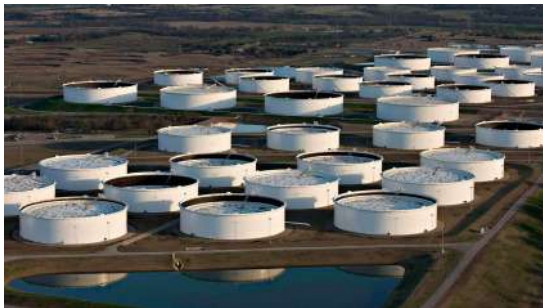
Floating Roof Storage Terminals
